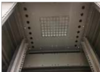
顶部出风孔焊接滤网 Filter on the top ventilation hole
