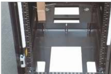
底部走线孔 Cable entrances on the bottom
